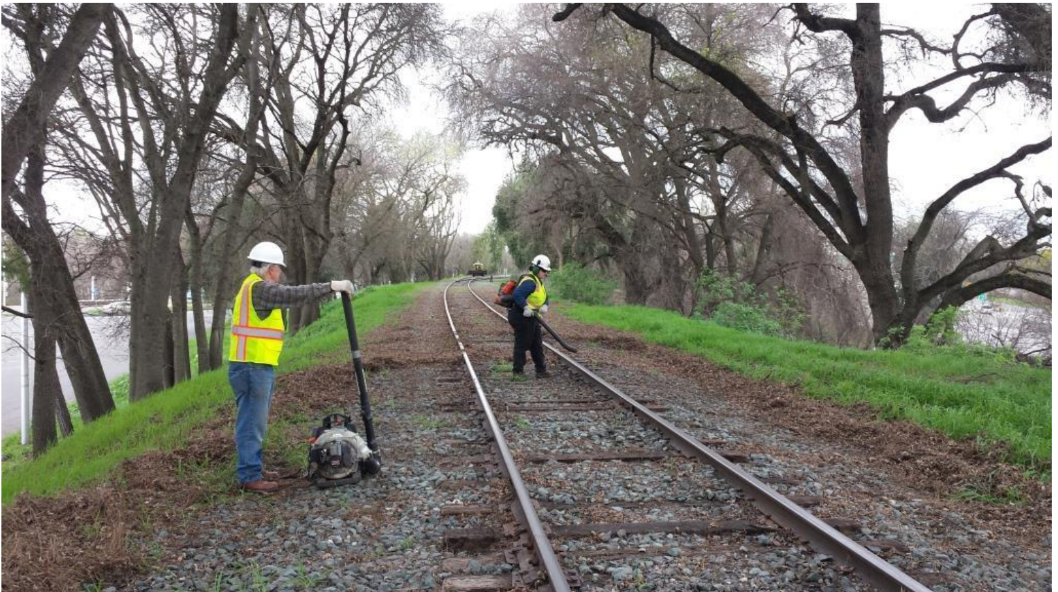
Mike W. and Heather use the wind machines to remove organic debris from the track
