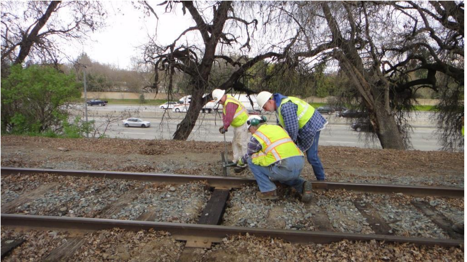
Steve put on a clinic on how to drive spikes using his patented “windmill” stroke. Here, he’s giving pointers to Mike M. while Mike H. nips the tie.
